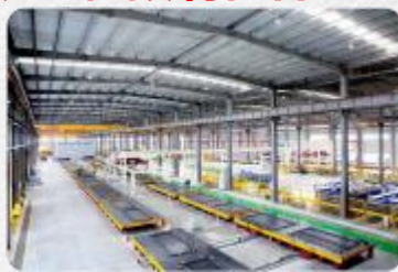
Carousel Plant 环形生产线
